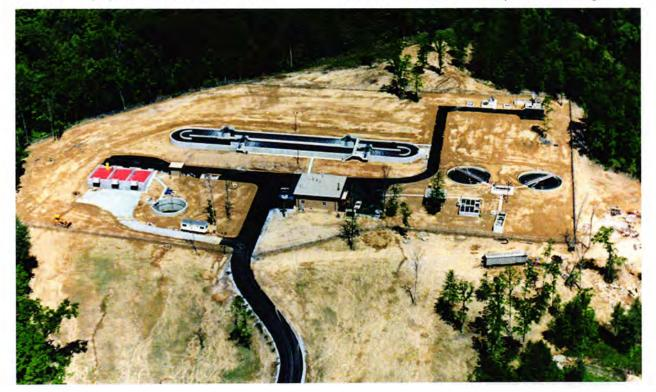
effluent standards established for the facility by the state. The new facility was designed to use the activated sludge process for biological removal of organic matter. The oxidation process was selected due to its ability to provide removal of carbonaceous biochemical oxygen demand and ammonia nitrogen in the same treatment unit. Also, the process is tolerant toward shock loadings and a relatively low power user compared to other processes.
