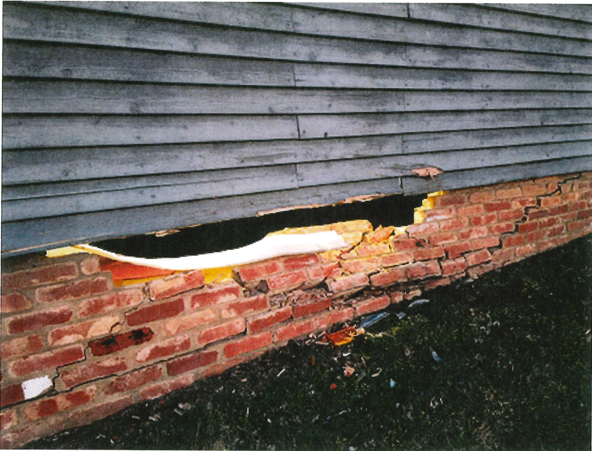
Image from car damage to existing barn on west side.
