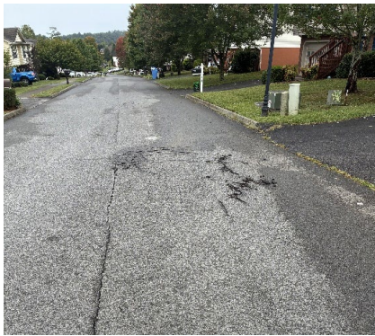
Meadow Creek Asphalt Degradation/ one of Several areas
