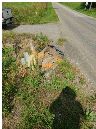
Old Boones Creek Main Drain Washout
