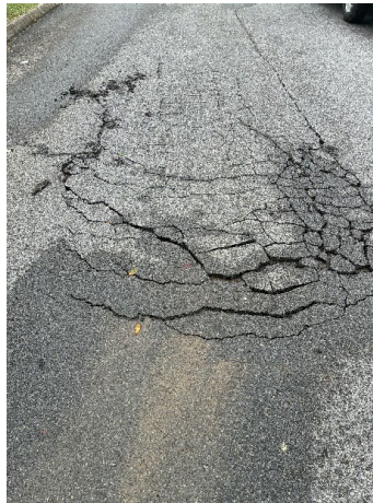
Meadow Creek Asphalt Degradation/ one of Several areas
