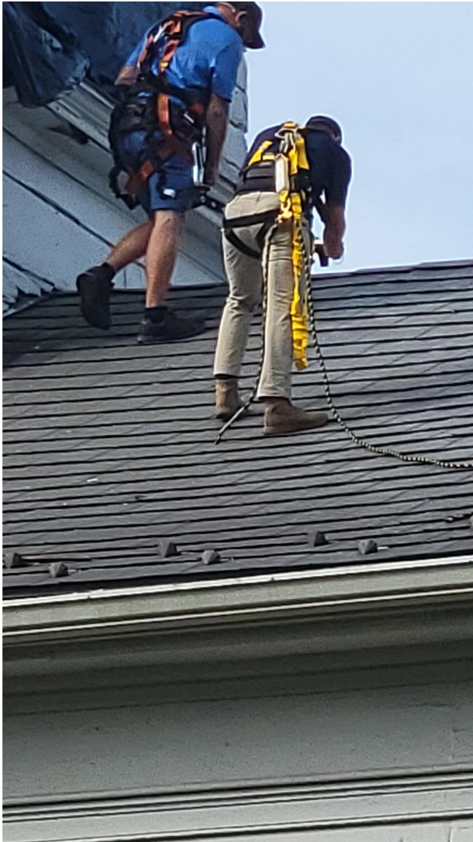
Photo 8: Structural Engineer and Building consultants hired by our Insurance to ensure repairs were done completely and correctly.
