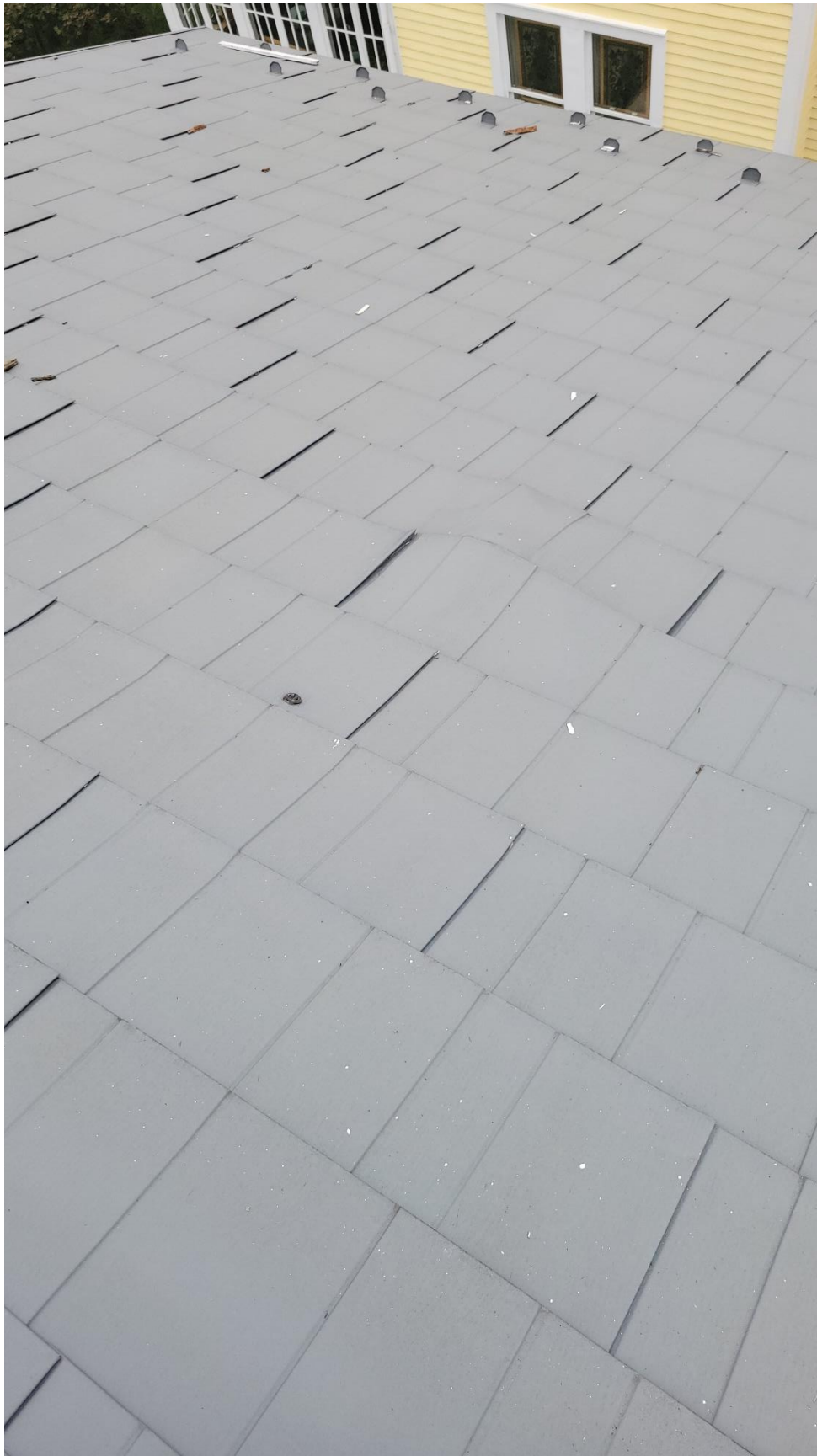
Photo 15: Another view of existing roof tiles.
